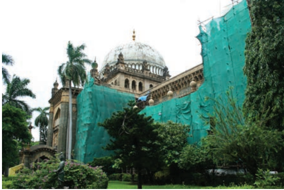
Building restoration in progress
