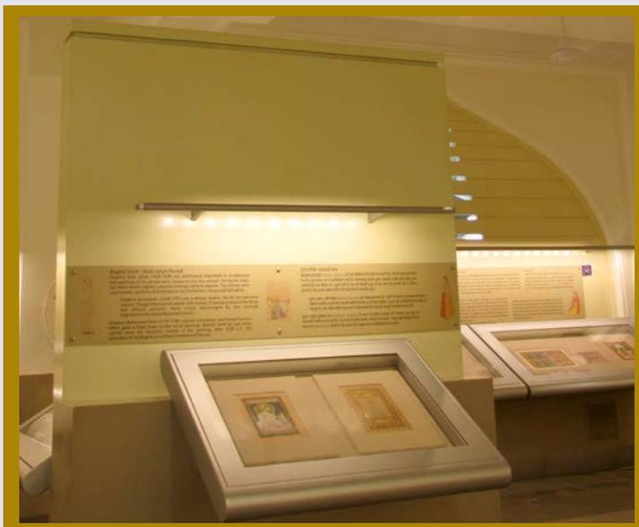
Lighting is one of the most important and difficult consideration in relation to the display of miniature paintings. It should be a perfect combination of good colour rendition and conservation friendliness. The required result of 50 lux and UV free lighting was acquired from specially ordered LED light bars. The problem of reflection was solved by adjusting the angle after several rounds of demonstration.
